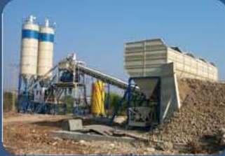
Saç İstinad Perdeli Bunkerler Aggregate Bunker with Reinforced Steel Retaining wall
