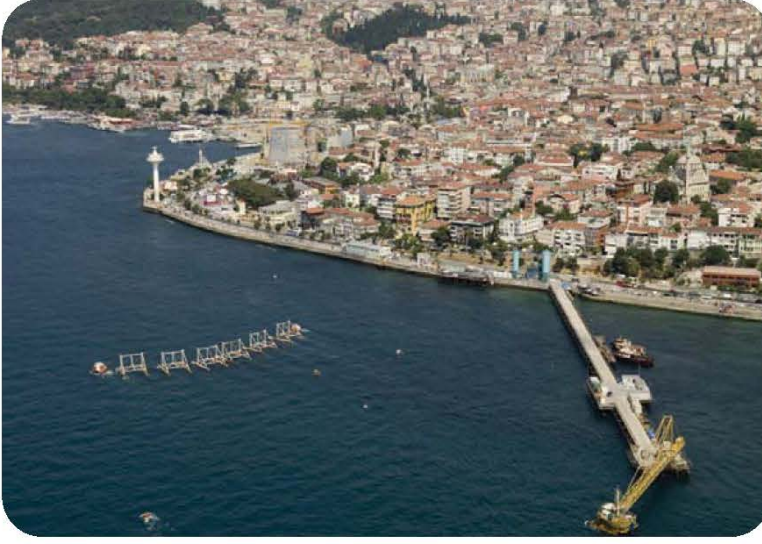
Marmaray Boğaz Tüp Geçiş Projesi Marmaray Railway Tunnel Under Marmara Bosphorus
